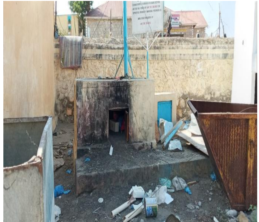
BRH Old incinerator
